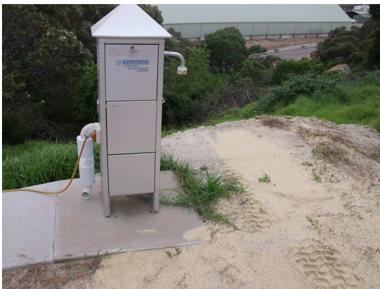
Figure 7. Earthworks carried out next to HVAS Site 3.
